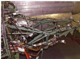
ABOVE Engine systems pipe work and electrical cables are refitted to the engine bearer. (Bruce Irvine)
