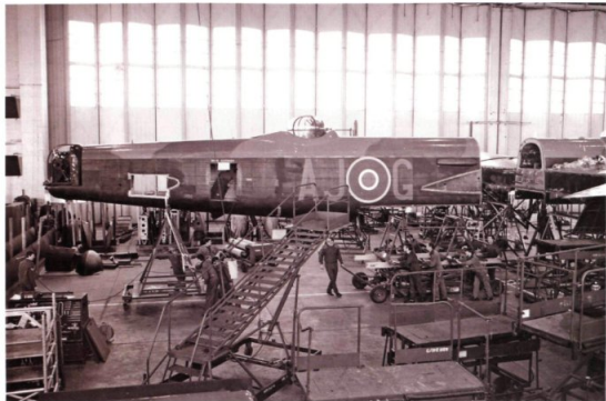
ABOVE Again seen at Abingdon in 1963, the Lancaster's rear fuselage has been separated from the centre section. Note that at the time it was wearing the AJ-G markings of Wing Commander Guy Gibson's ED932 from the famous 'Dam Busters' raid. (Crown Copyright)
